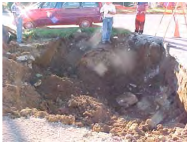
Excavation of Underground Storage Tank
