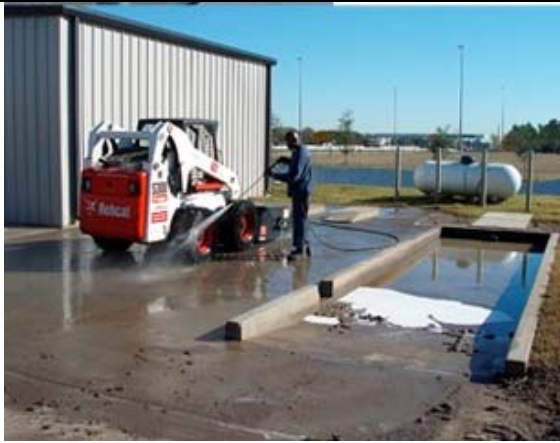
Clean trucks and equipment in the designated location.
