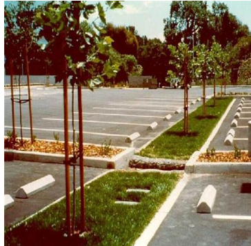
Rain Gardens, Bio-swales & porous pavements allow for infiltration of runoff
