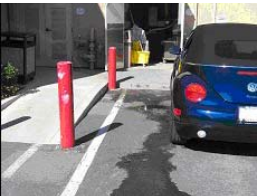
Non-Stormwater flows into storm drains (illicit discharges) are easily found during periods of dry weather
