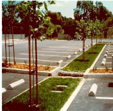
Bio-swales & porous pavements allow for infiltration
