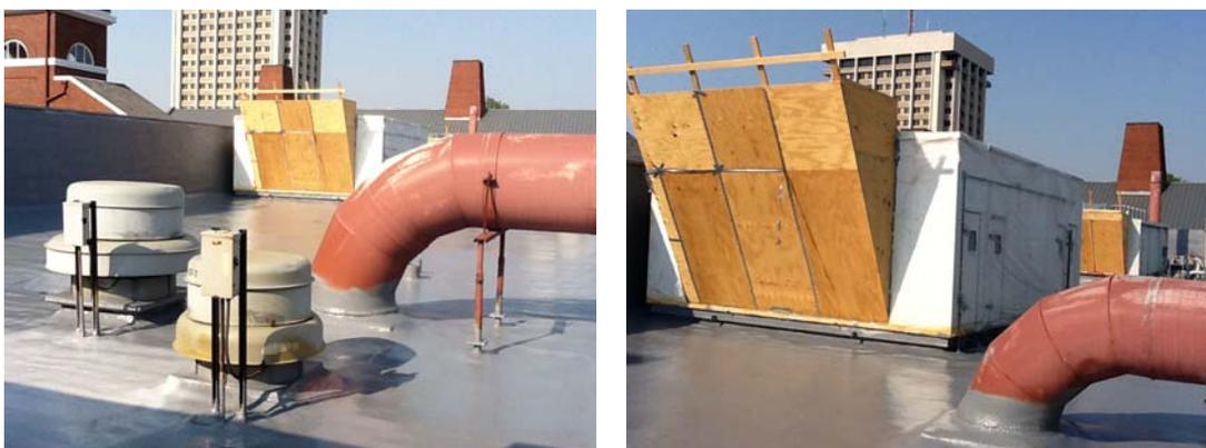
*Photos above show rooftop following application of Basecoat. Modifications to air intake (wooden deflector, doors sealed with plastic sheeting) are visible.*
